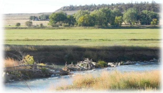
Figure 2. High flows flanked this rock riprap now sitting in the middle of the channel adding to the overall stability problems. Photo Credit: K. Boyd.
