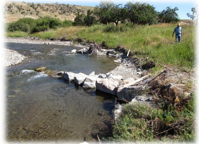
Figure 3. High flows can damage properly installed bank protection treatments when the system is not in balance. This weir and bioengineered bank will require maintenance for some time into the future. Photo Credit: T. Pick.
