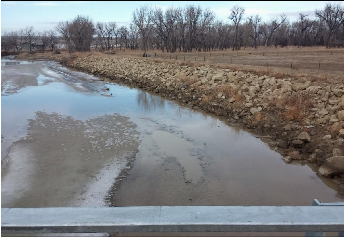
Figure 46. View downstream from 2 nd Street Bridge showing rocked berm on right bank at Roundup Fairgrounds, February 10, 2015.
