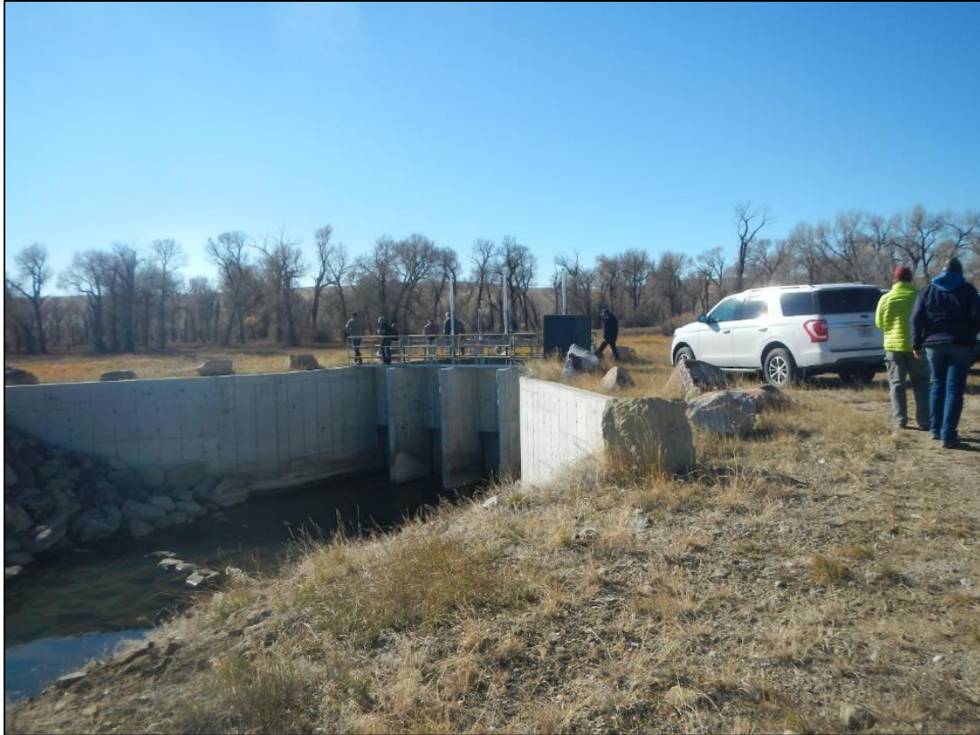
Figure 5. Reconstructed headgates at Deadman's Basin Diversion Dam (2021).
