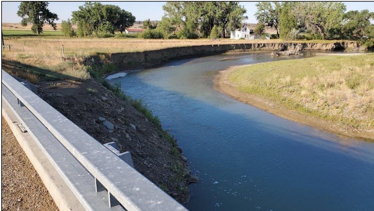
Figure 45. View upstream from the Cushman Road Bridge showing right bank erosion and current stabilization efforts, August 9, 2021.
