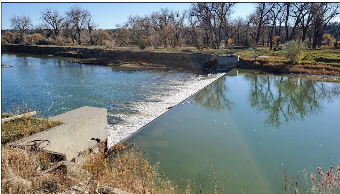
Figure 48. Kilby Butte diversion dam, November 1, 2021; a bypass channel has been proposed around the diversion on the far side of the river.
