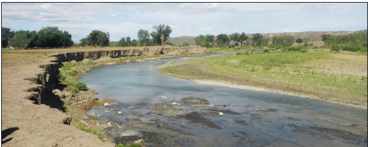
Figure 63. View downstream of eroding left bank selected for preliminary design of erosion control.
